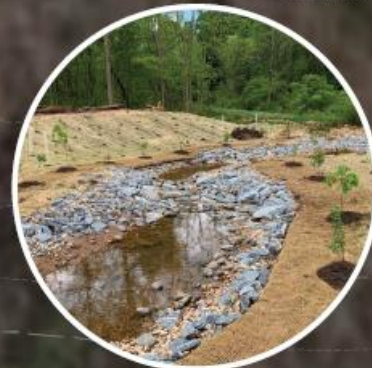
Example Gully Repair
