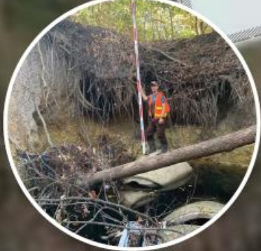
Existing Pipe Outlet
