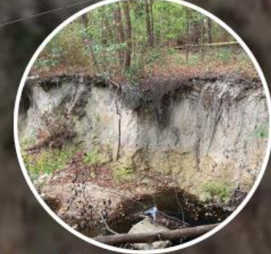
Existing Stream Bank Erosion
