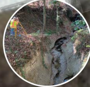
Existing Stream Bank Erosion
