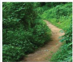
Compacted Earth Trail 3'-0" wide
