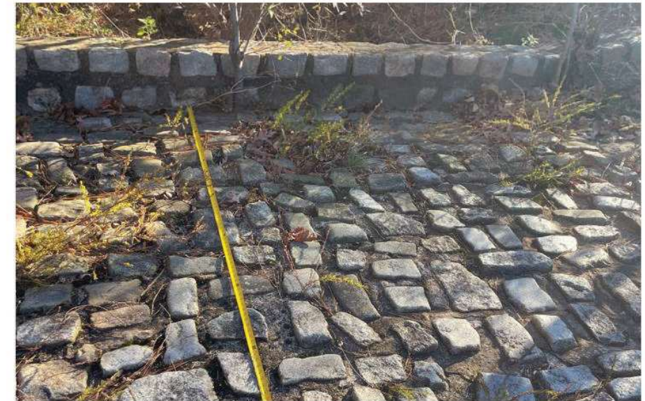
EXISTING MATERIAL - COBBLESTONE SPILLWAYS
